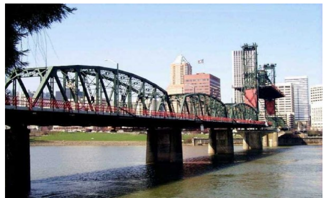
Hawthorne Bridge, looking into downtown Portland
